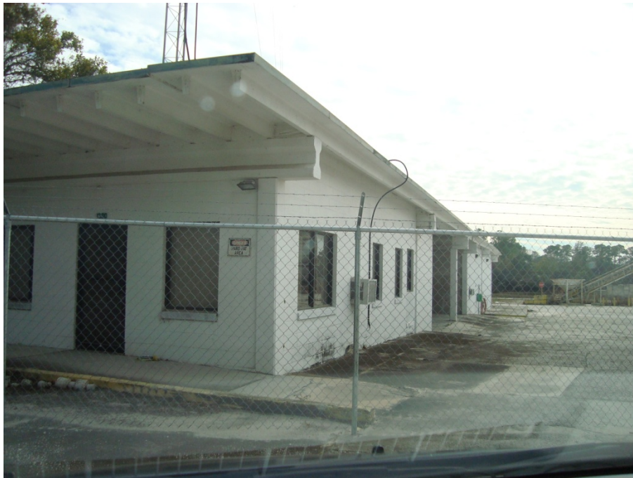
Offices at temporarily shut-down facility (Cemex – 0690003).
