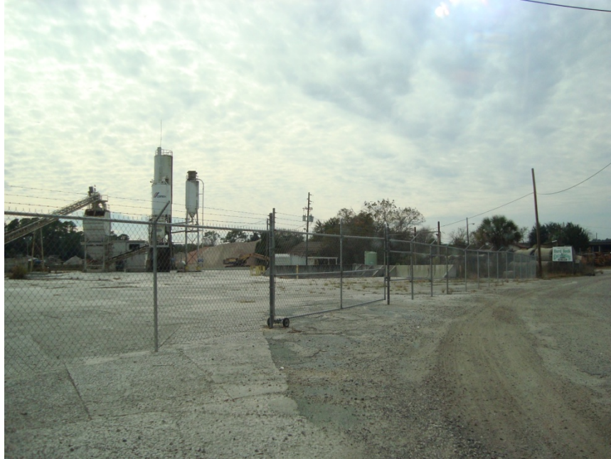
Front gate locked at temporarily shut-down facility (Cemex – 0690003).
